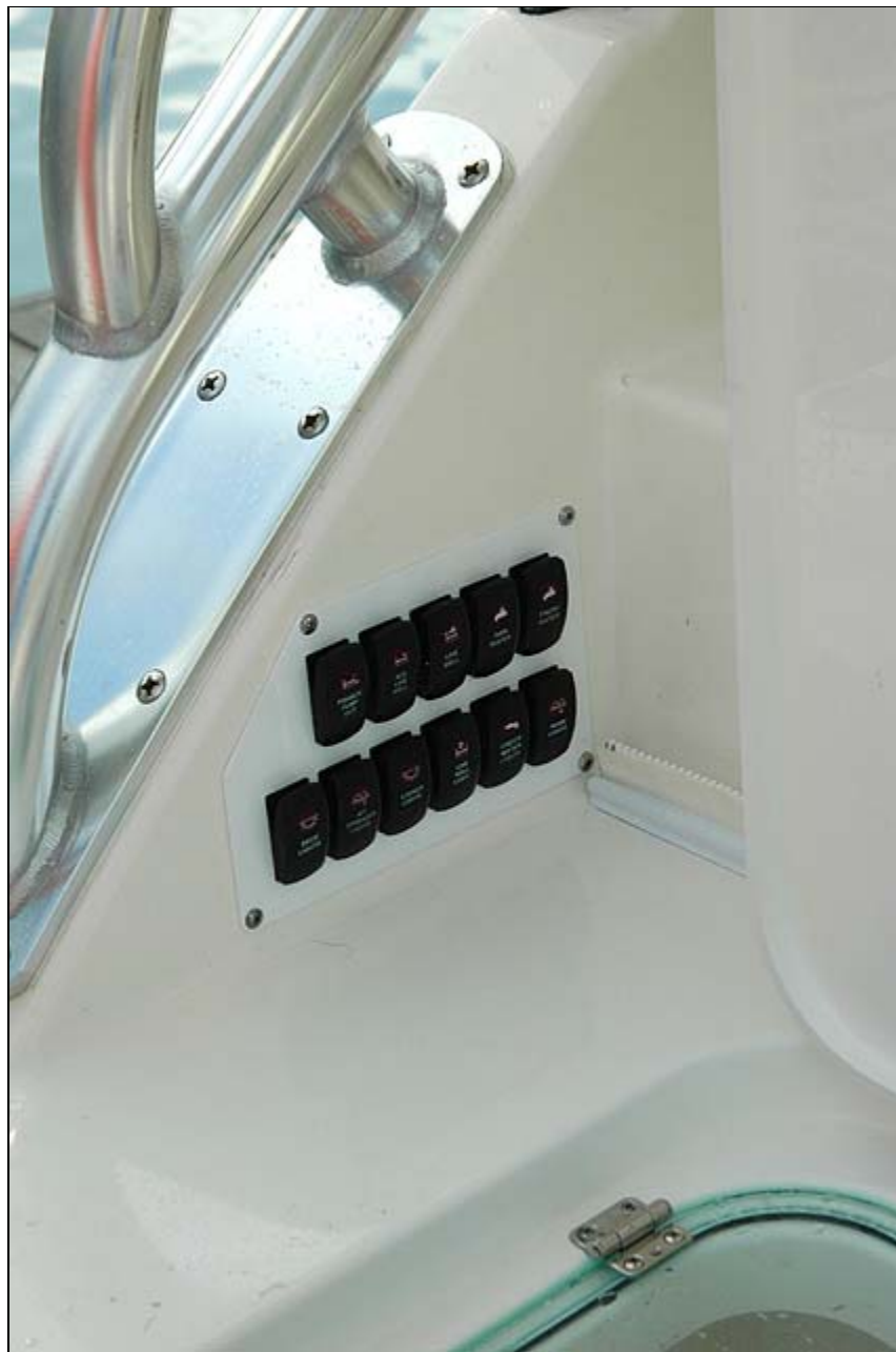
All of the switches for features like lights and wells on the helm panel are also on the instrument panel in the cockpit right above the livewell, for quick access.
